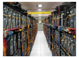
The most common method used for controlling data center cooling devices employs the return air temperature from the data center. This method provides a blended air temperature regime from the data center to the cooling devices that masks the actual needs of the servers. Consequently, the cooling devices will operate inefficiently because they do not accurately anticipate cooling requirements.
